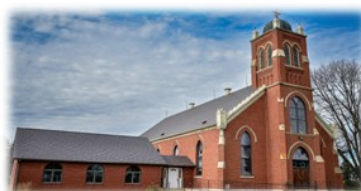
St. Columbkil Church (SC) 36483 County 47 Boulevard Goodhue, MN 55027
